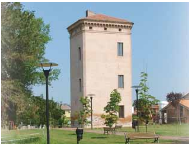
La Torre (sec. XVI) • The Tower (16th century)
