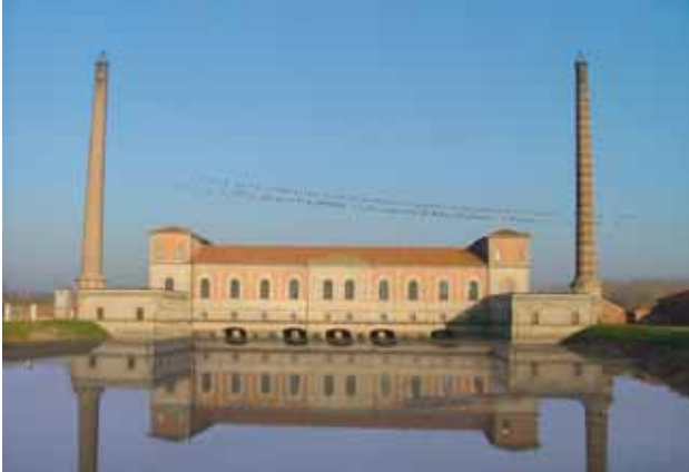
Bonifica Agro Mantovano-Reggiano (sec. XX°) • Draining installation "Agro Mantovano-Reggiano" (20th century)
